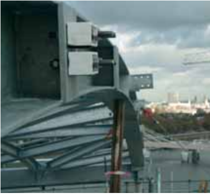
Steel beam with Schöck Isokorb® type KST
