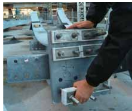
Fitting a Schöck Isokorb® type KST to a steel beam
