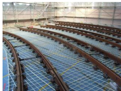
Floor slab Tram Depot Basel, CH 2009
